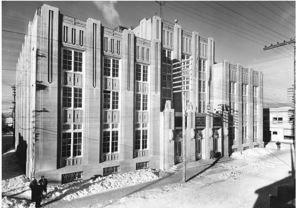
The current Old Federal Building, was completed in 1934. ( https://www.fjc.gov/history/courthouse/fairbanks-alaska-1933 Source: National Archives, RG 121-BS, Box 3, Folder H, Print 2 (ca. 1933))
