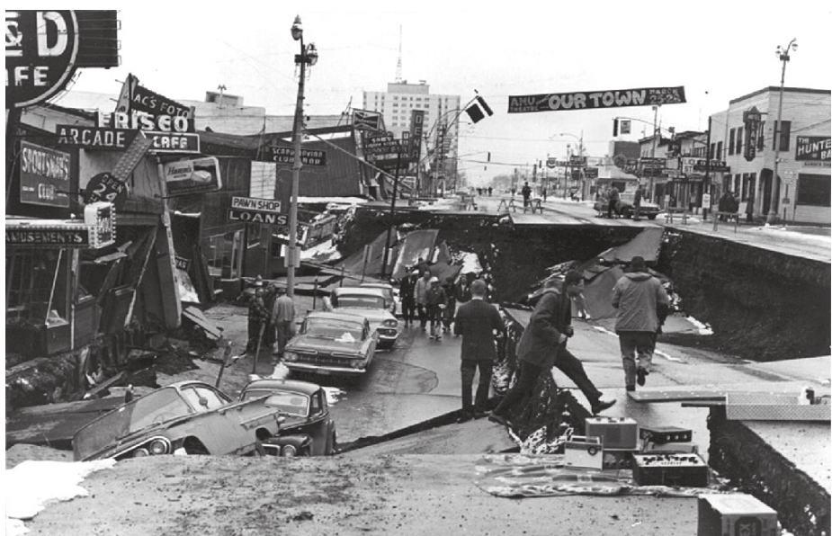
Earthquake damage: Fourth Avenue looking east. Google Images
