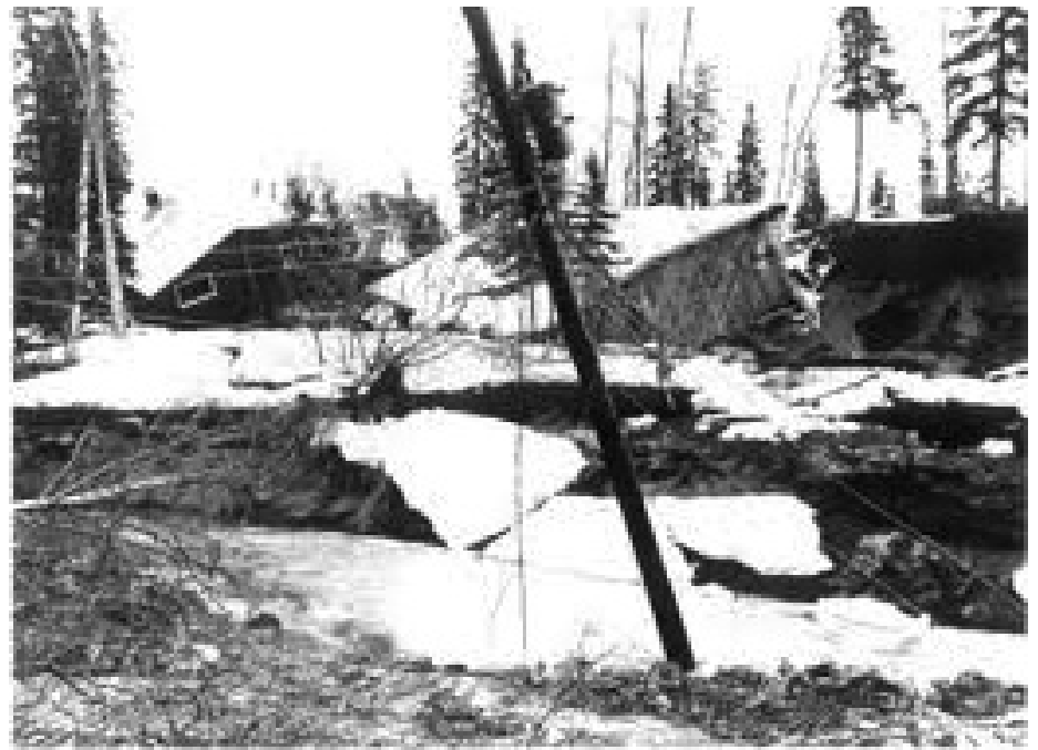
Subsiding land collapsed under homes in Anchorage's Turnagin subdivision. (USGS photo)
